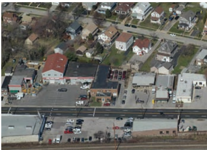
Wide Curb Cuts Should be Narrowed to Provide Increased Safety and Pedestrian Orientation along Haverford Road
