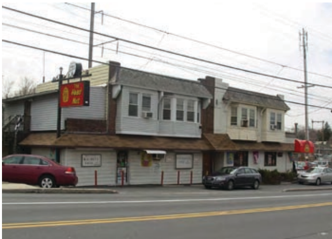
Apartments Above Commercial, Haverford Road
